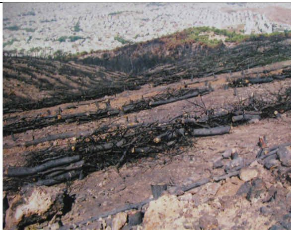
Figure 7. Detail of the log-barriers built constructed immediately after the Kareas fire (shown in Figure 6) immediately after their construction.
