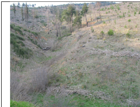
Figure 5. Branch piles along the contours and a log-dam in a ravine, built in the forest-park of Thessaloniki, Greece after the fire of July 1997. Photographed here in 2004.
