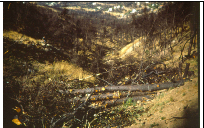
Figure 10. A check-dam constructed with logs in a ravine on Penteli mountain, within 3 months after the 1995 fire.
